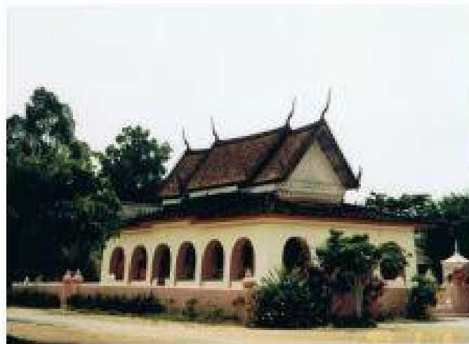
Figure 02. Ubosot of Wat Machimmaram before renovation Source: Khoruamdetch (2013)
