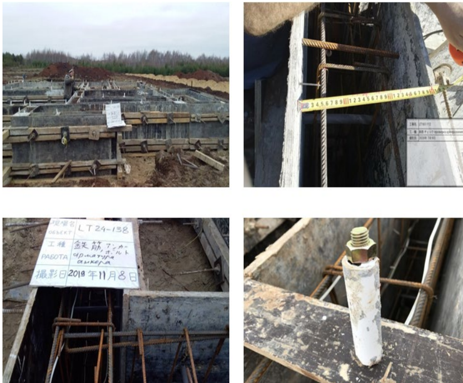
Figure 4. Inspection of reinforcement, installation of formwork, anchors
